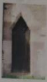
The design of the Chancel door with the sharply pointed arch is believed to indicate a pre-Norman date.
