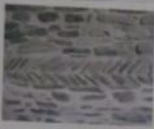
The 'Herringbone' masonry in the lower part of the north wall of the Nave
