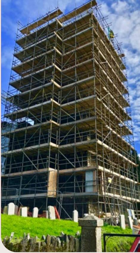
Repairs to St Julietta, Lanteglos by Camelford, Cornwall
